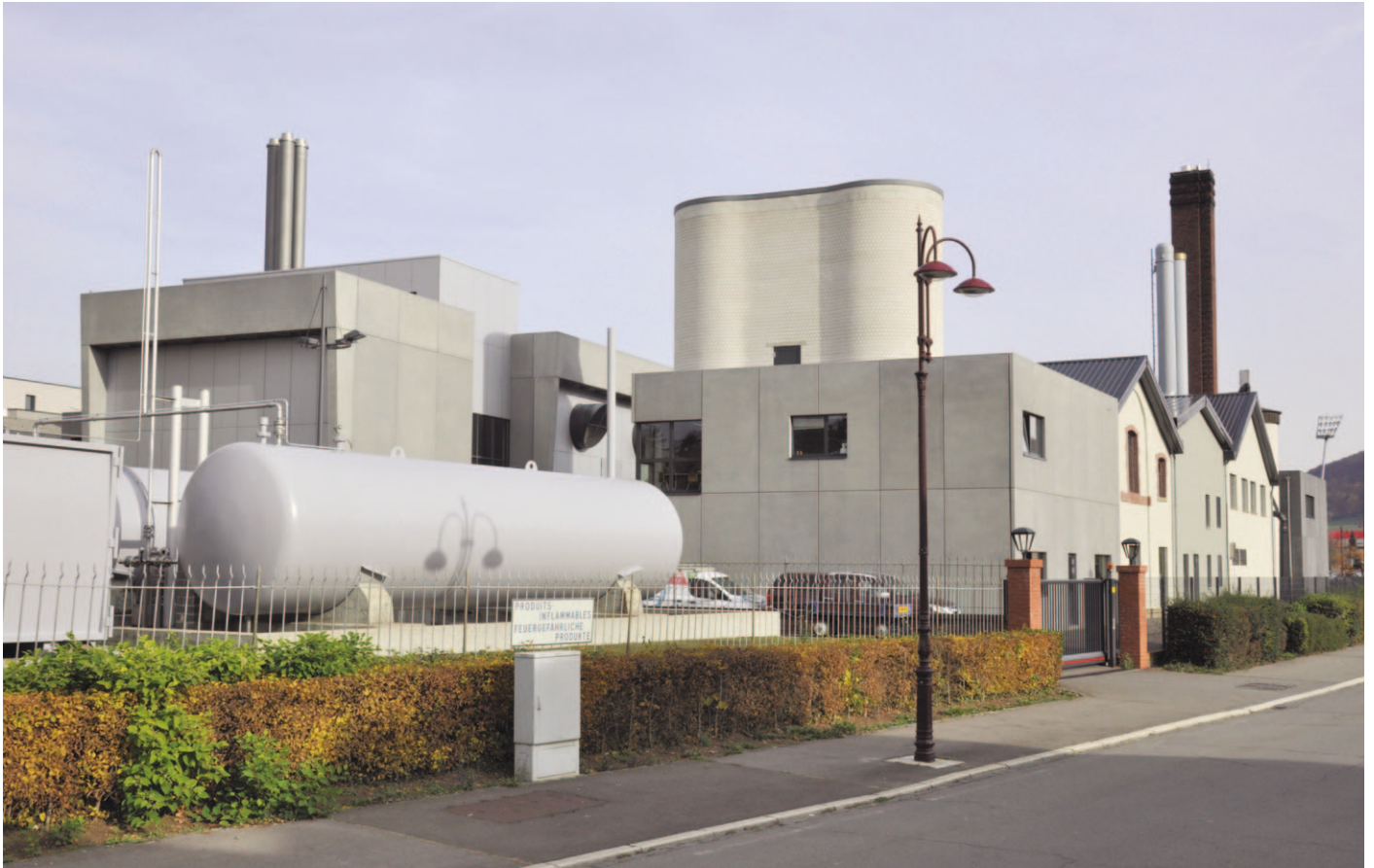
Site Services Industriels no Renovatioun
