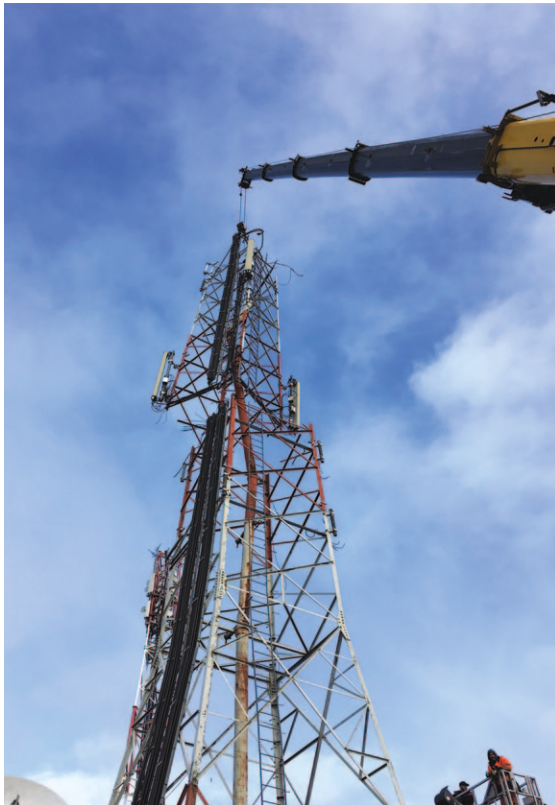
Demontage alen TV Mast
